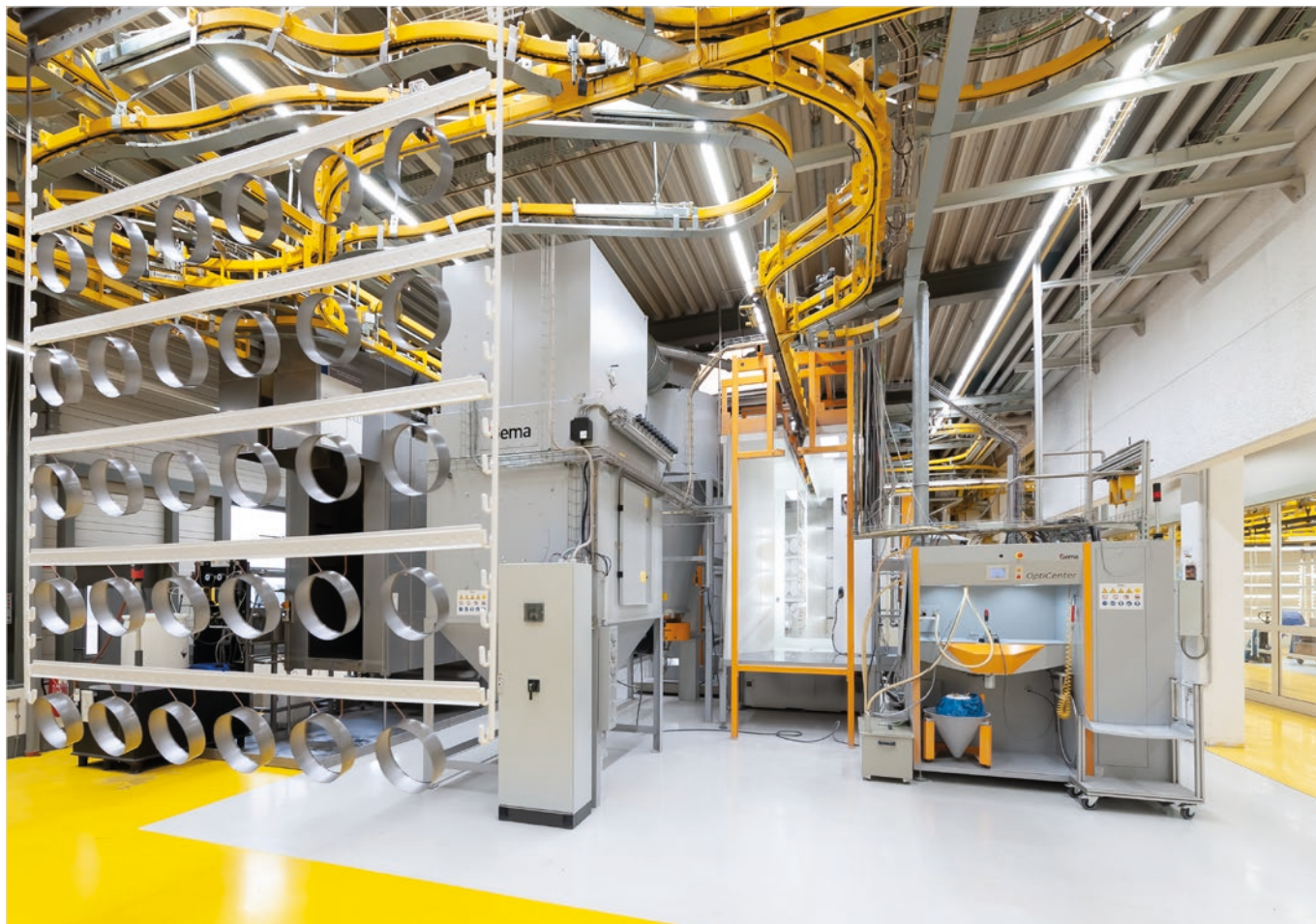
Installation de thermolaquage
